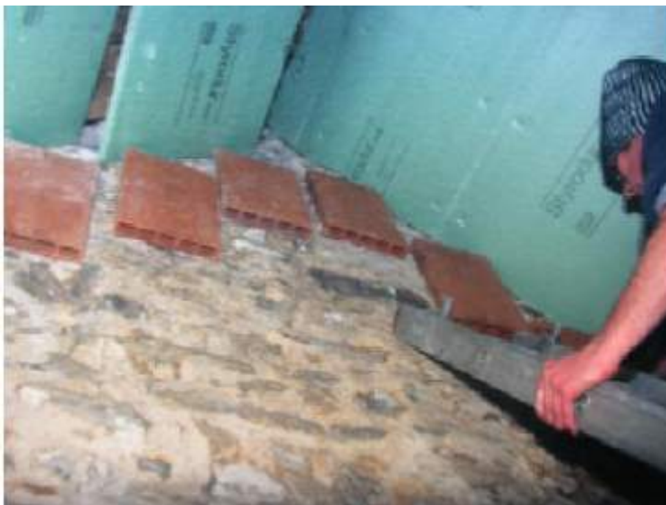
Figure 18: installation de briques (source GMB)
